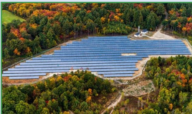
**Description:** The solar farm is situated on approximately 10 acres of land surrounding one of the water district's pump stations and is interconnected to existing electrical infrastructure that serves pump station equipment on site.
